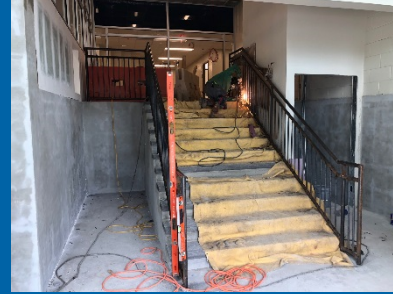
Installing Handrails at Main Entry Stair
