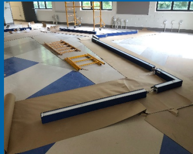
Installing Custom Light Fixtures at the Stem Lab
