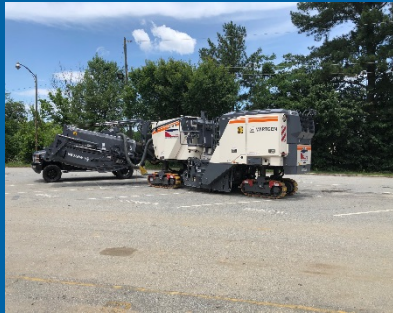
Paving Equipment Delivered to the Site
