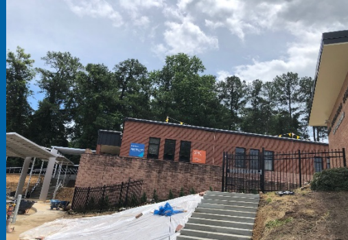
Installing Decorative Fence, New Site Stair, and Grading of the Site
