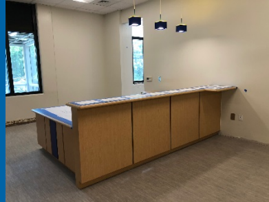
Finish Install of Casework at Entry Admin Area
