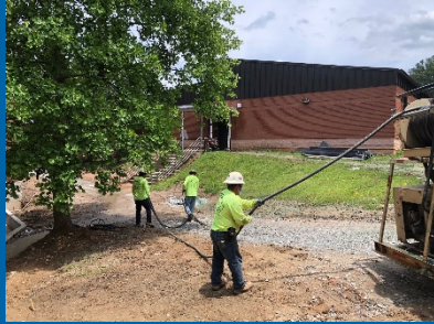
Hydroseeding the Site
